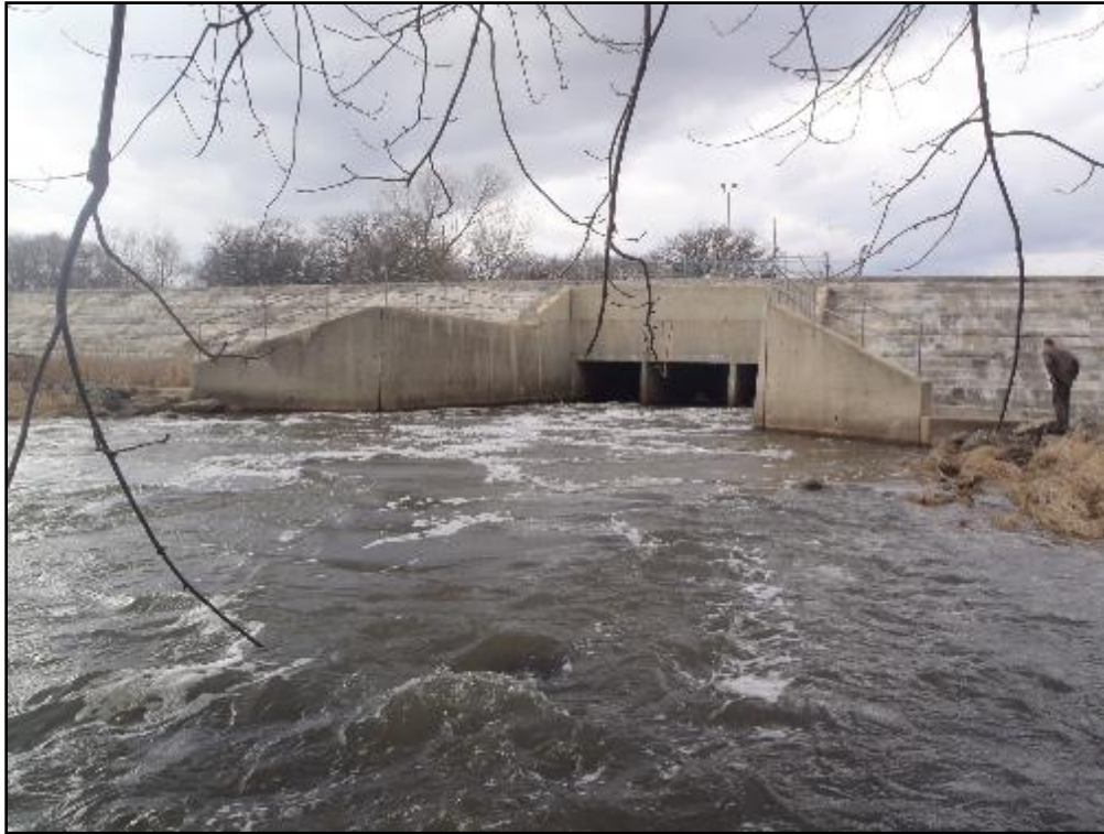
Plate 3. Fawell Dam viewed downstream of the dam looking north towards the dam. The three-culvert system is visible in the center of the photograph.
