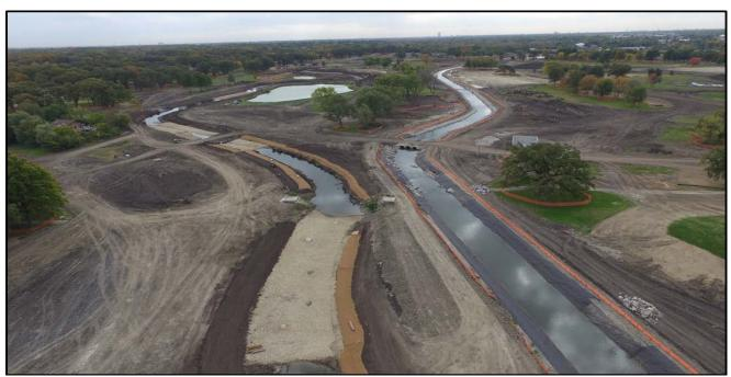
**Figure 2**. The view (south) from the diversion dam at the upstream end of the project (near Elizabeth Drive) prior to flow being reintroduced to the engineered channel. The diversion channel is at the right of the project area. The restored river channel is on the left of the image with exposed gravel runs/beds and graded stream banks still under construction.
