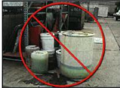
How NOT to store materials Outdoors, in leaking containers
