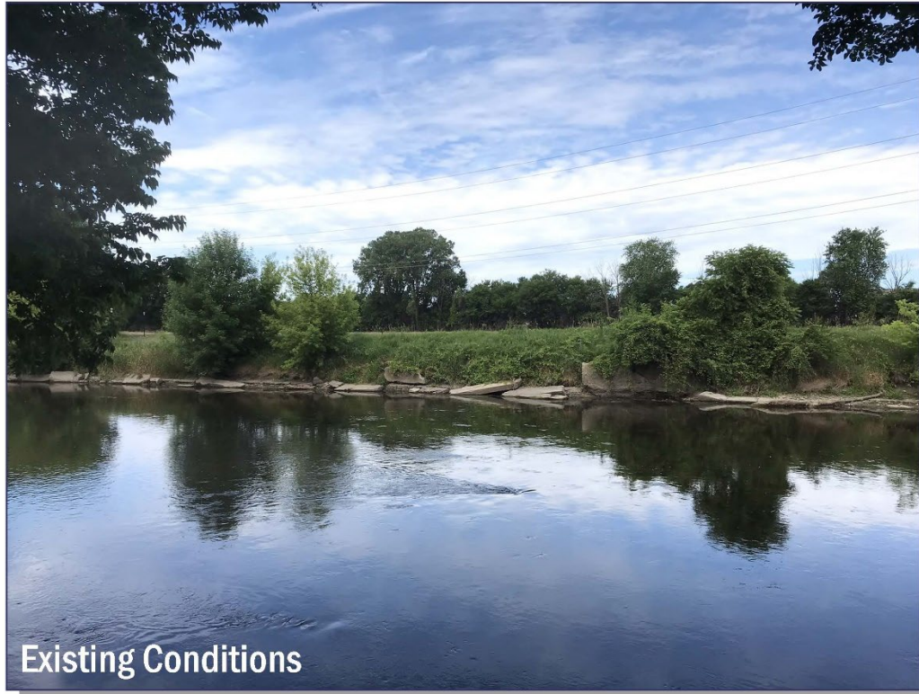
Lower DuPage River - Failed Wall and Bank Stabilization
